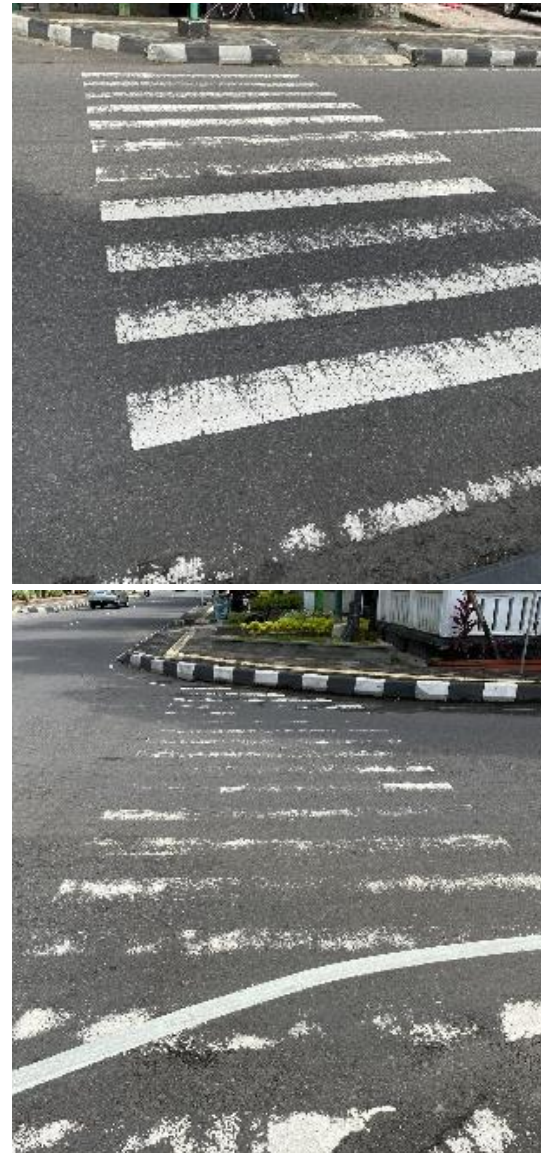
Figure 5. Crossing facilities on the Parasamya street corridor
