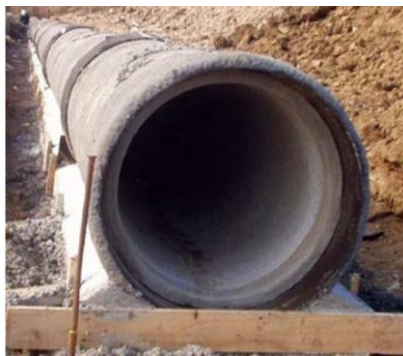
Figure 1. Precast concrete conduit: (a) schematic (b) installation [2]
